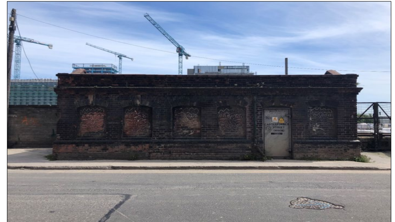
Figure 4.5: Detached single storey electricity substations external to the site on Castleforbes Road. Source: TPA, May 2020. Collated by TPA, January 2021.
