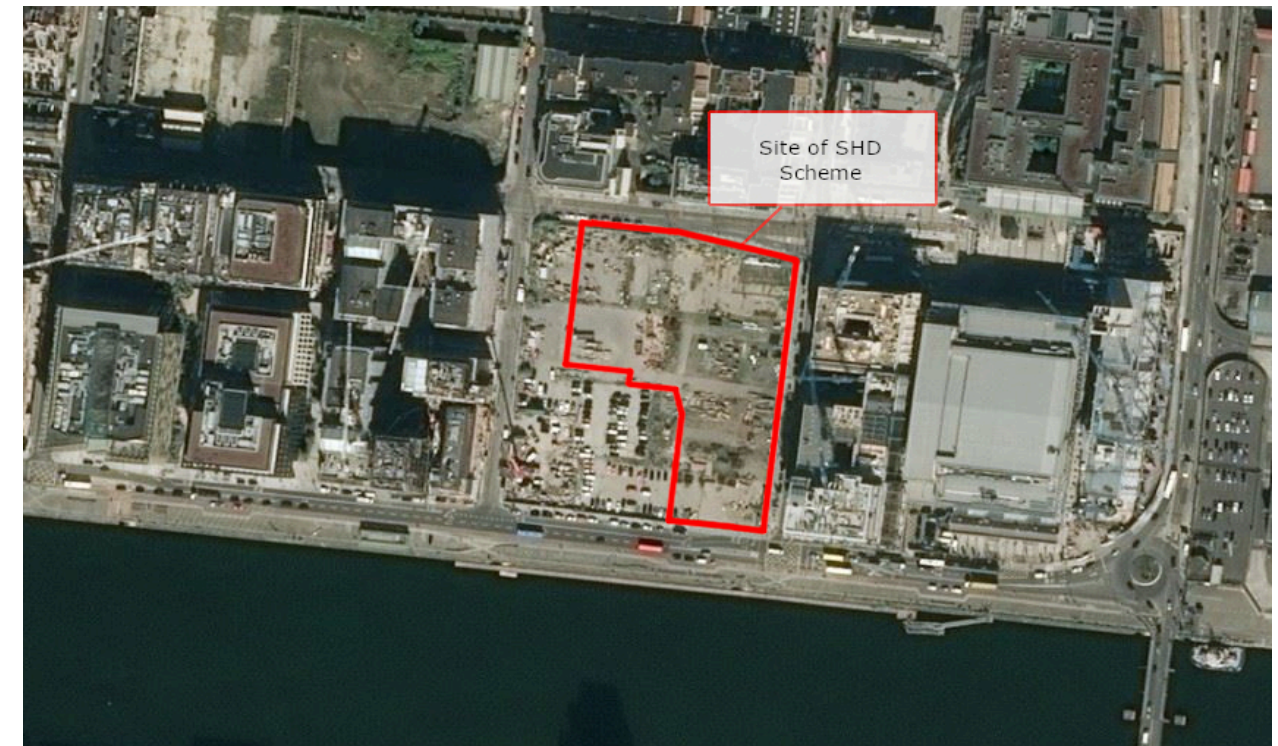
Figure 1.1: Aerial photo showing the indicative boundary of the Subject Site outlined in red, with the balance of the City Block 9 outlined in blue. Source: Bing. Cropped and annotated by TPA, January 2021.
