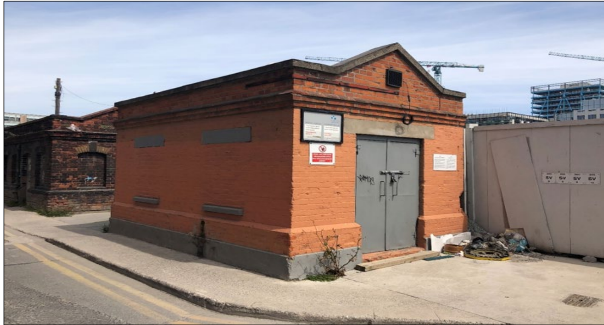
Figure 4.6: Detached single storey electricity substations external to the site on Castleforbes Road. Source: TPA, May 2020. Collated by TPA, January 2021.
